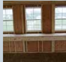
32" Workbench 2" x 6" framing
