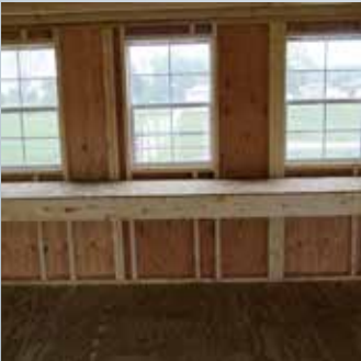
32' Workbench 2" x 6" framing
